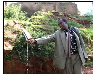
Headmaster Ombati shows how the water tank works. The partially-submerged water tank is the large concrete structure in the back.
