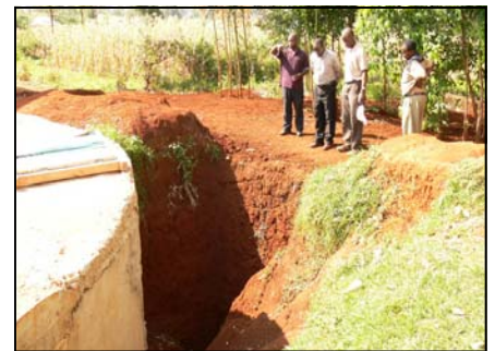
Inspecting the Ritaro tank
