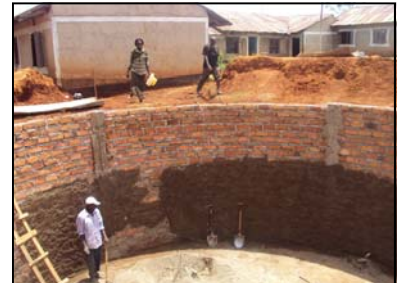
October 2009 - Finishing walls
