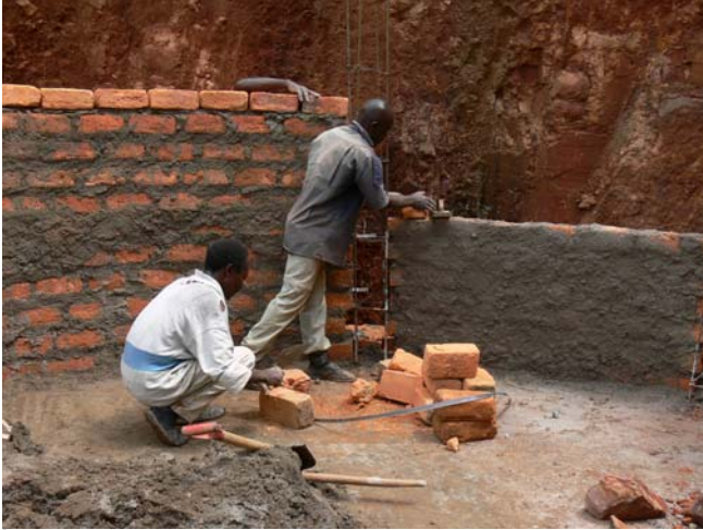
Construction of Water Tank at Boruma School
