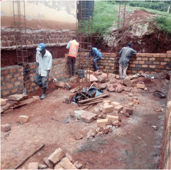
Erecting brick walls
