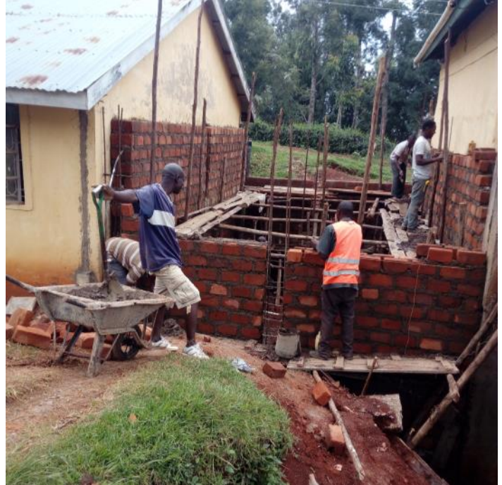
Brick work continues
