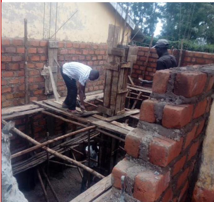
Working on concrete supports
