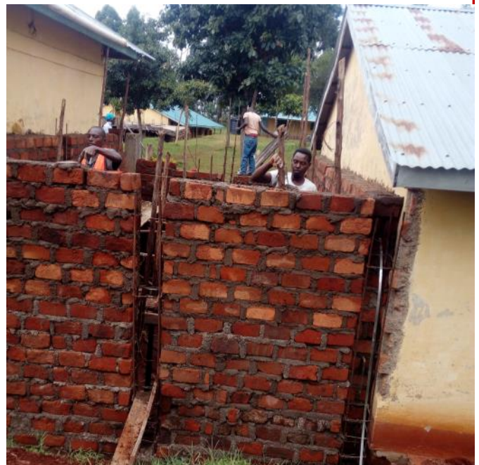
Brick walls nearly complete
